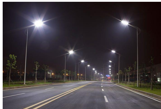
View of Assembly Street lighting project
