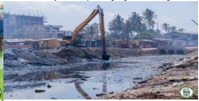
Ongoing desilting of drains in Accra
