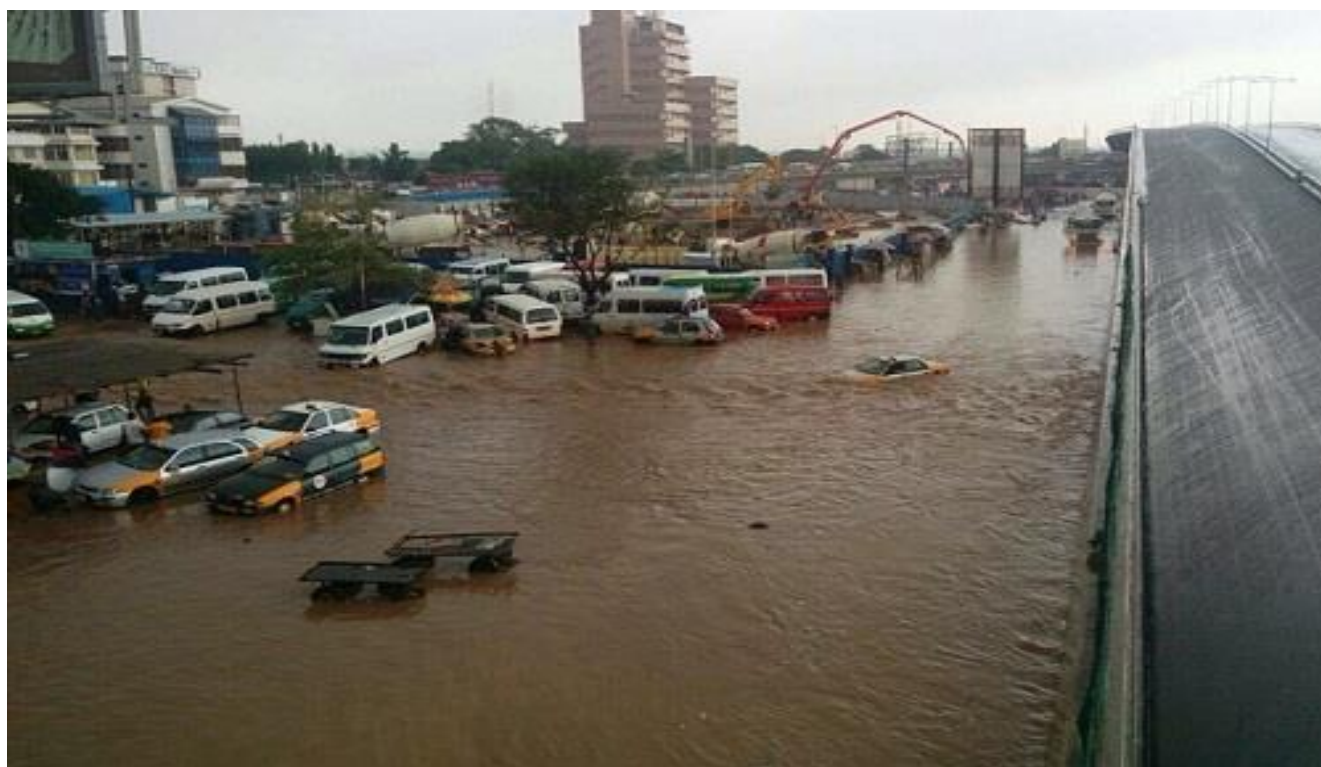
Part of the city flooded during a rain storm in June 2016
