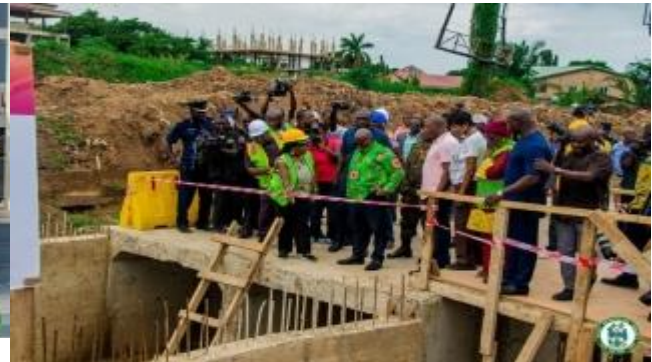
President Akufo Addo inspects ongoing works to mitigate
