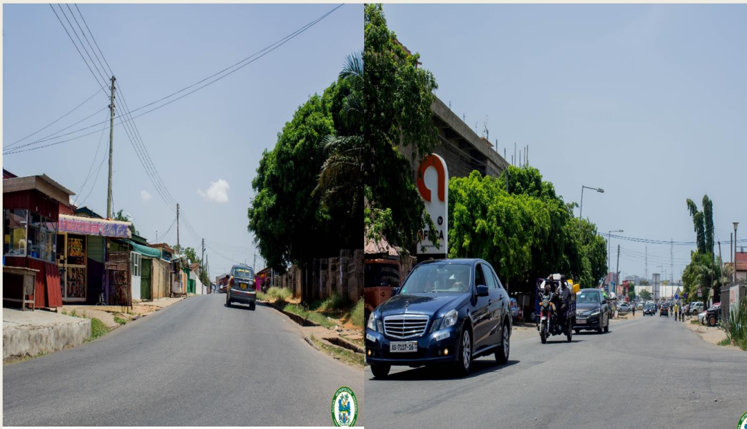
ASPHALT OVERLAY ON AZUMA NELSON STREET
