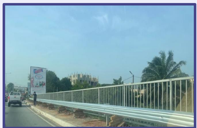
Installed crash barriers along Olusegun Obasanjo Highway
