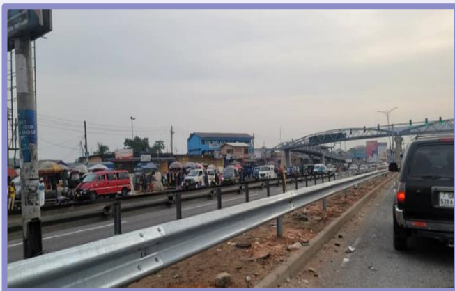
Installed crash barriers along Lapaz section of the George Walker Bush Highway (NI)
